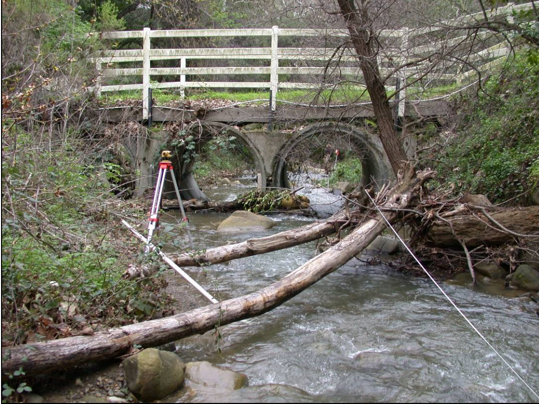
Figure 4 - Inlet of Lower Crossing, consisting of three 7-foot diameter concrete culverts.
