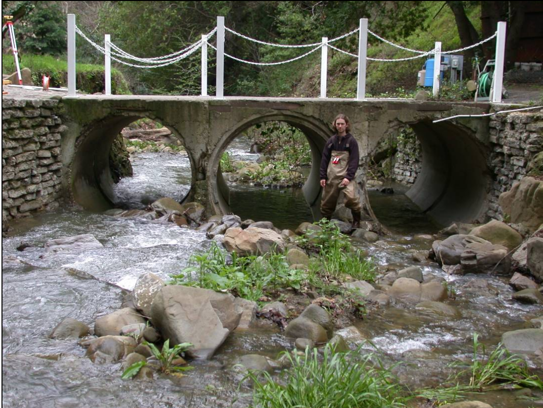
Figure 5- Inlet of Upper Crossing, consisting of three 6-foot diameter concrete culverts.
